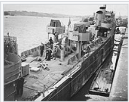
HMS Campbeltown being converted
